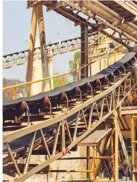
COAL HANDLING PLANT AT NORTH KARANPURA
