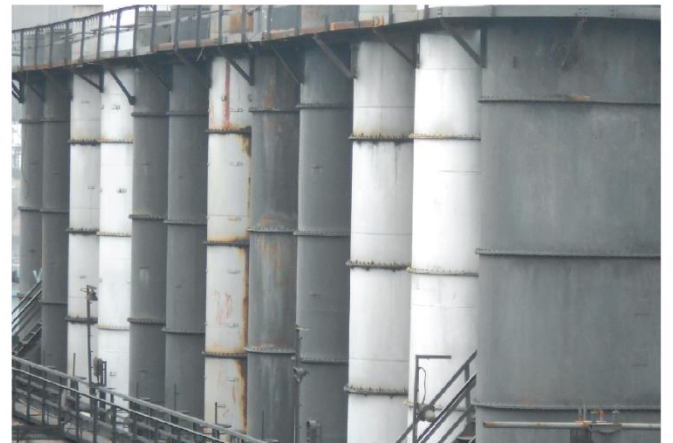
SAIL, DSP PRIMARY GAS COOLER
