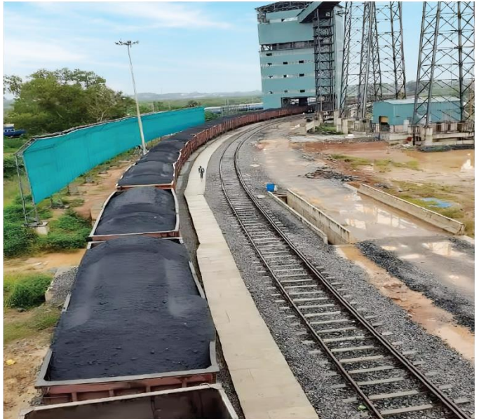
COKE HANDLING SYSTEM WITH RLS & PIPE CONVEYOR AT MRPL
