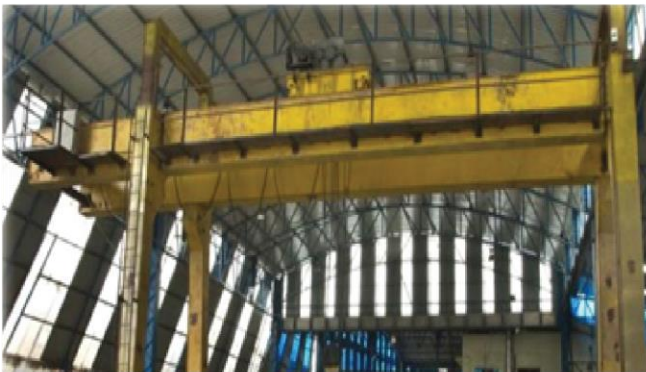
GOLIATH CRANE (HANDLING MATERIALS)
