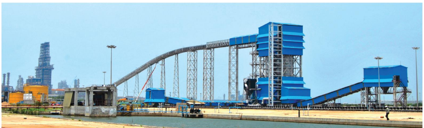
PET COKE HANDLING SYSTEM IOCL AT PARADIP
