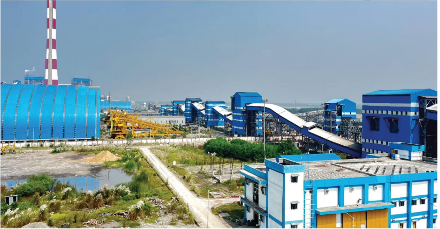
COAL HANDLING PLANT FOR BHEL BANGLADESH MAITREE (BIFPCL)
