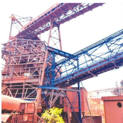
NEW CRUSHER BUILDING AND ASSOCIATED CONVEYORS PLANT AT SAIL BOLANI
