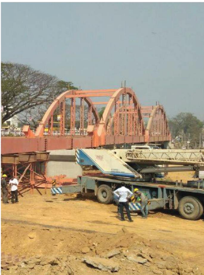
FABRICATION & SUPPLY OF STEEL ARCH BRIDGE FOR NCC AGARTALA, KATAKHAL FLYOVER PROJECT
