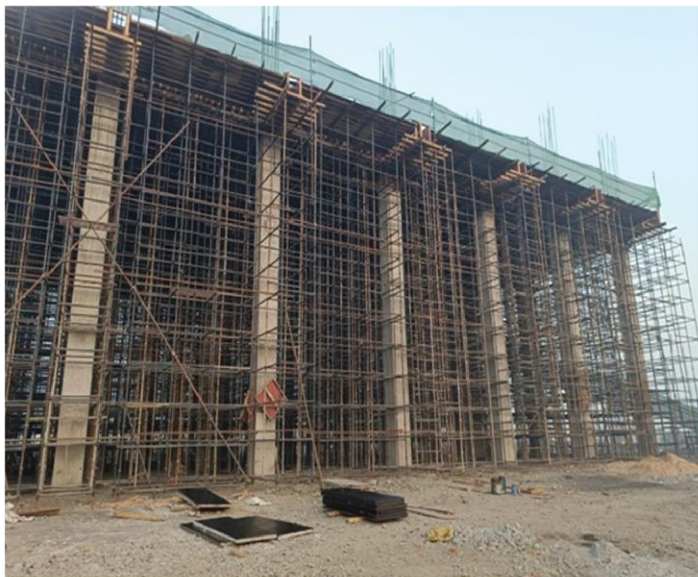
UREA HANDLING & BAGGING PACKAGE AT TFL, TALCHER
