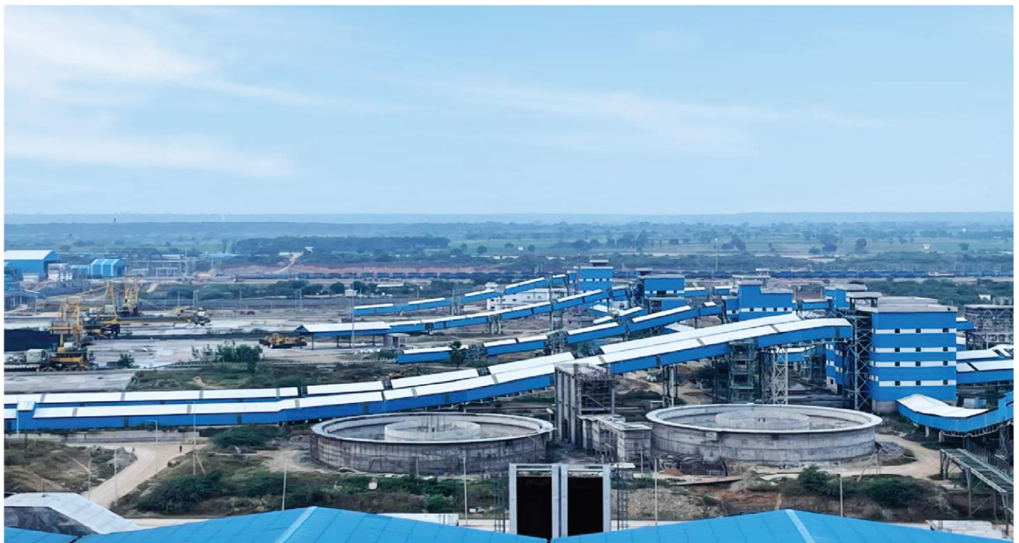
COAL HANDLING PLANT AT YADADRI - 5X800 MW
