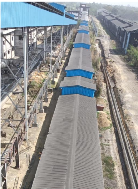
COAL HANDLING PLANT AT NBPPL, UNCHAAR
